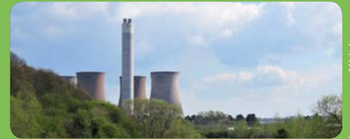
Demolition of Rugeley Power Station began in 2019
