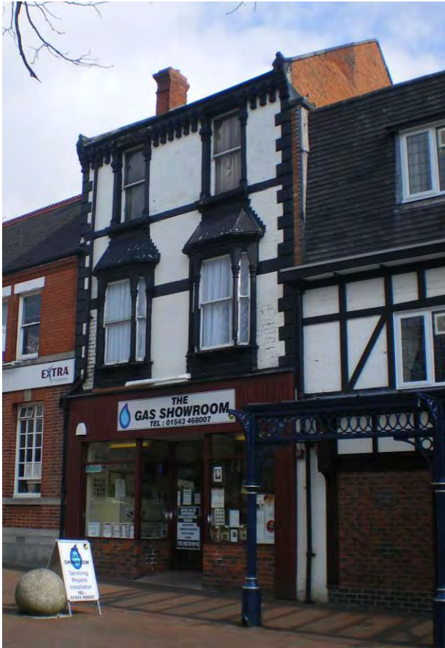
Plate 7: Surviving burgage plot north of Market Place
