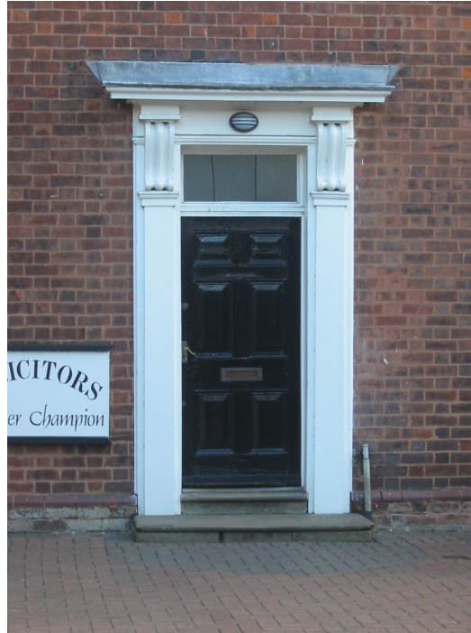
Fig. 2 Door case at Brook House
