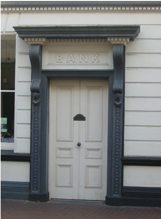
Fig. 3 Door case 16 – 18 Lower Brook Street
