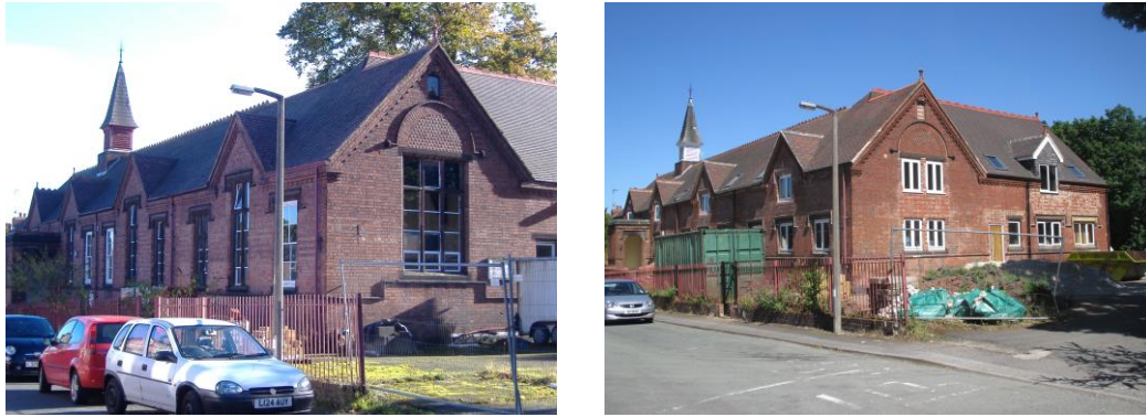
Fig. 4 The former Talbot Street School, before and during conversion to residential use.
