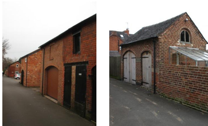
Fig.3 Coach houses rear of Talbot Street properties
