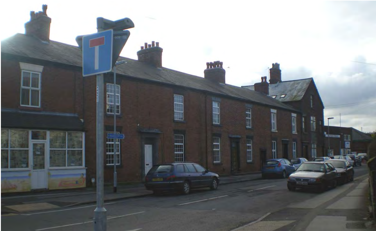
Plate 12: 19th century properties in Market Street
