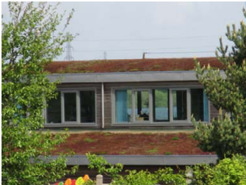
Green Roof at Chasewater Innovation Centre provides a wildlife habitat
