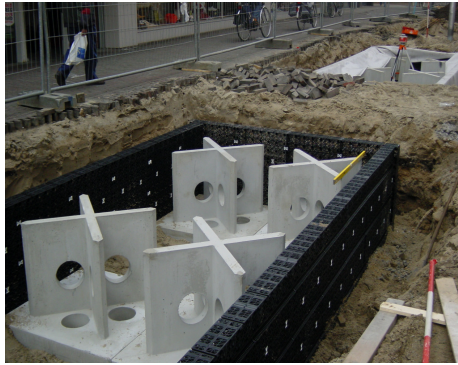
Root box constructed under paving
