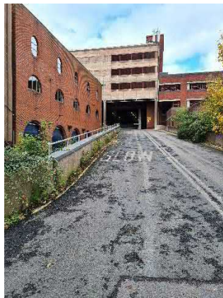
Photograph 7: Ramp to the closed multi-storey car park
