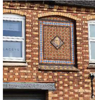
Photograph 2: Building Detail on Market Street
