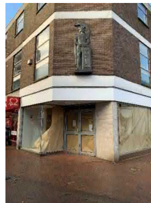
Photograph 7: Vacant unit at the corner of Bees Lane and Lower Brook Street
