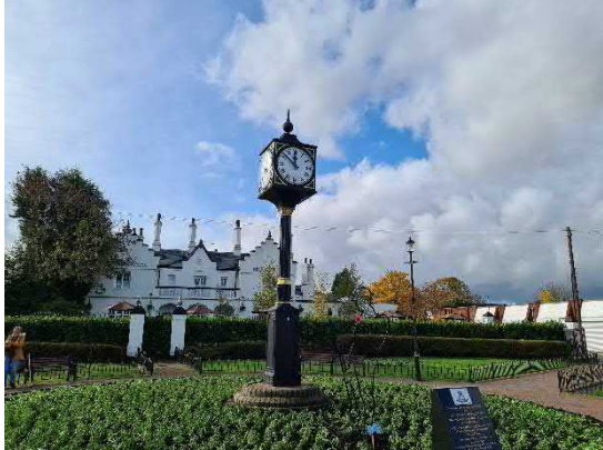
Photograph 1: Clock Tower and Anglesey Lodge
