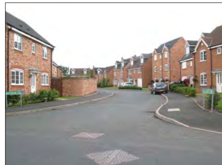
A different brick has been used at Littleton Green to create some variation but continual use has created too much repetition and lack of variation
