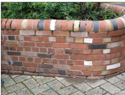
Brick walls used for raised planted beds and seating, with variation in brick colour
