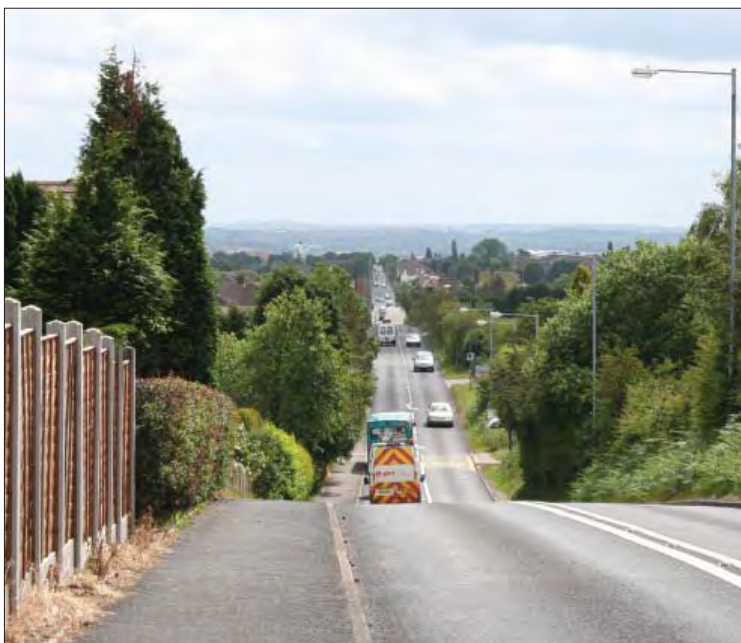
View down Pye Green Road
