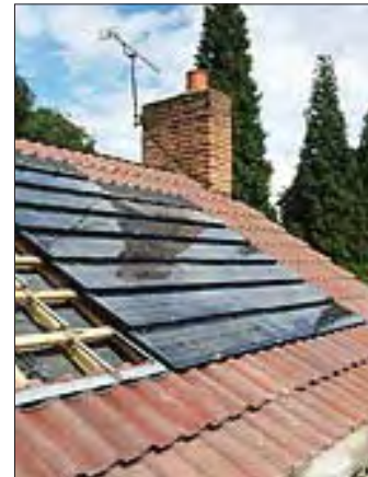
Solar panel installation
