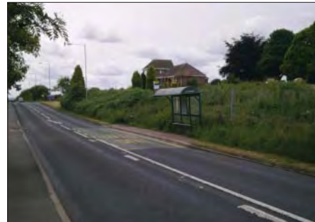
Existing bus shelter at the site
