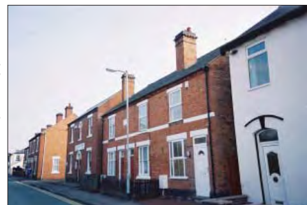
Victorian housing in Cannock in predominantly red and painted brick. A key feature is the white window sills and heads, window frames, and doors
