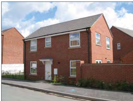
A typical detached house at Fallowfields, Huntington, in red brick with white features. This is again typical of many recent developments through-out the region and is not locally distinctive
