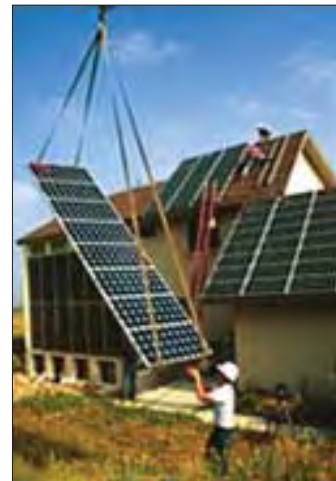
Solar panel installation
