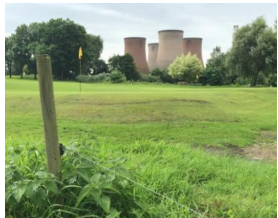
Figure 2.3 Existing Site (View of Cooling Towers from Golf Course)
