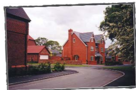
Speed restraint achieved by speed control bend. Please note that a mountable hard shoulder is required in certain locations - Dickens Heath
