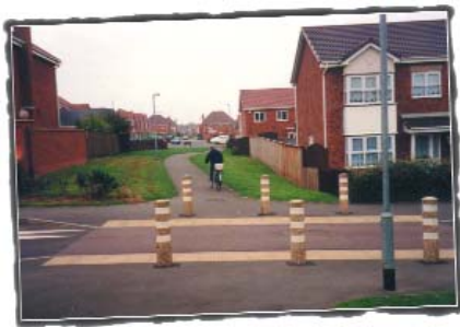
Safe cycleway crossing combined with speed controlling devices - Tamworth
