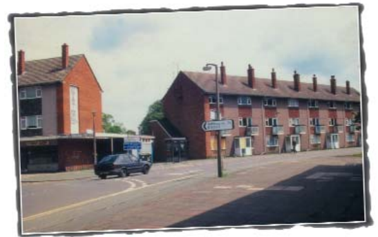
The existing site
