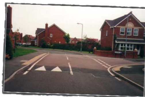
Tactile paving combined with speed controlling device to provide safe crossing points - Tamworth.
