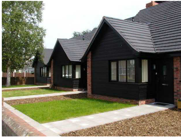
Fig.3 New almshouses at junction of Church Street and Fortescue Lane
