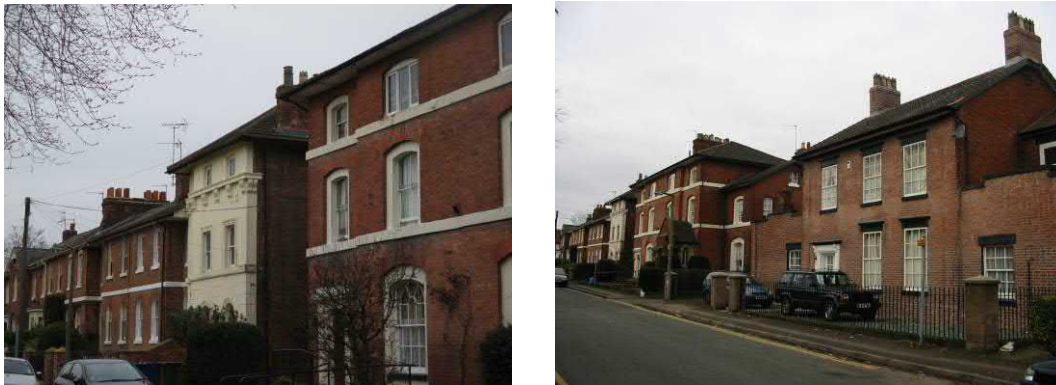
Fig.2 Villas and townhouses at 30-40 and 26 Talbot Street
