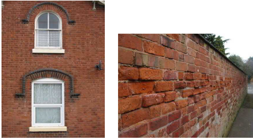
Fig. 14 Comparison and original and replacement upvc windows; decay of a brick boundary wall
