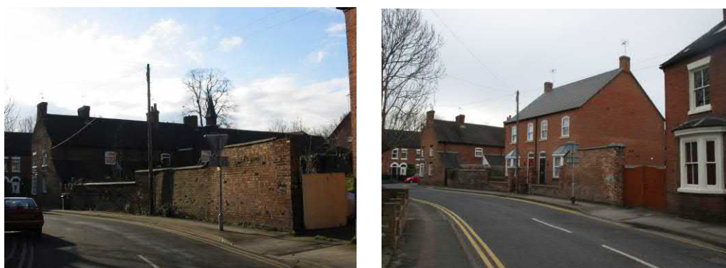
Fig.10 Adj to 52 Lichfield Street (before and after development)
