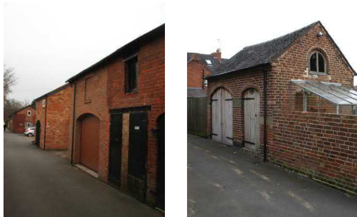
Fig.3 Coach houses rear of Talbot Street properties
