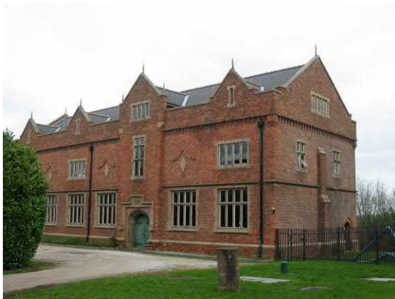
Fig. 1 Brindley Bank Pumping Station
