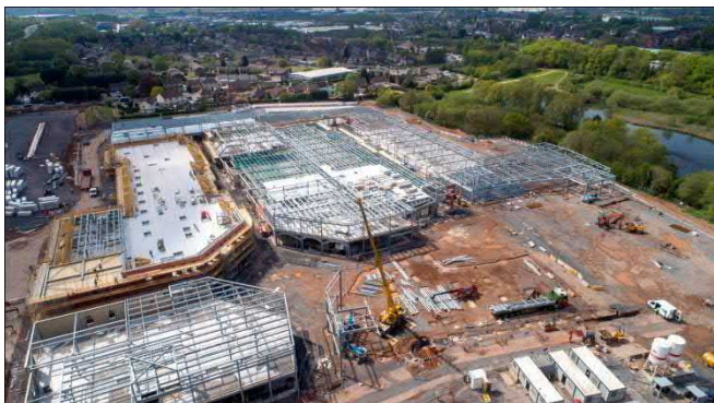
Steelworks for McArthurGlen Designer Outlet nearing completion
