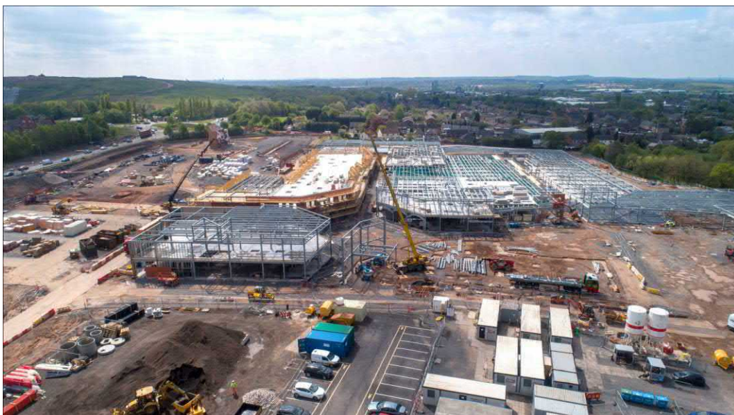
Taking shape – the McArthurGlen Designer Outlet retail complex in Cannock due to open in 2020.
