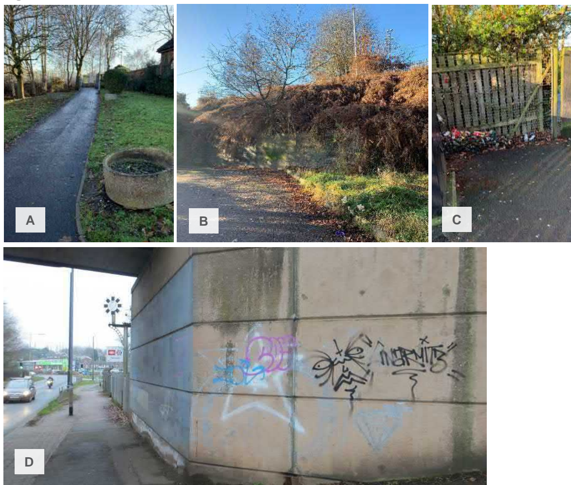
Figure 2-12 - Unattractive Features of the Current Cannock Station.
