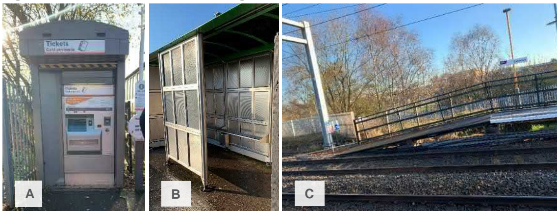
Figure 2-6 - Additional Photos Showing Basic Facilities at Cannock Station
