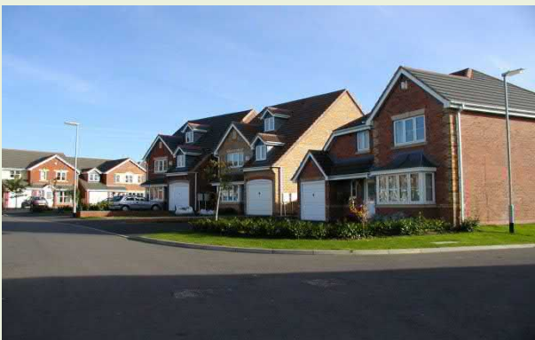
Modern Houses, Wimblebury
