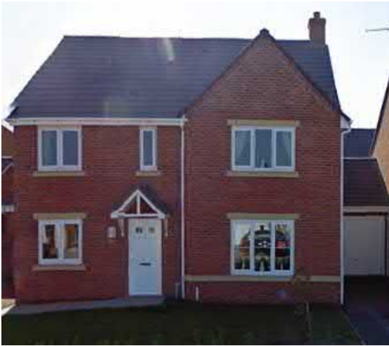
Figure 2.11 Example of surrounding residential development
