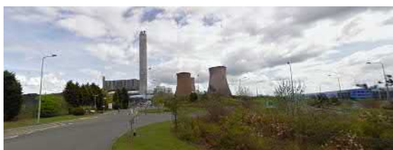
Figure 2.4 Existing site access from A51
