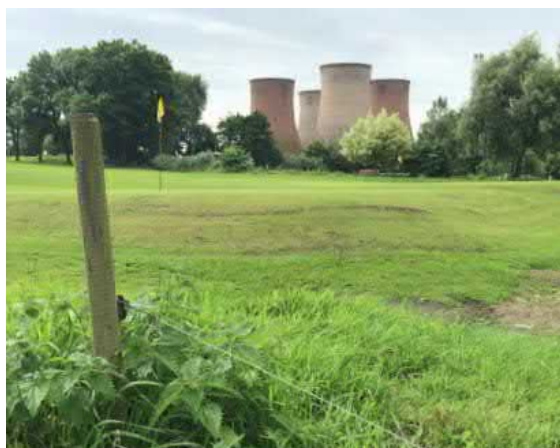
Figure 2.2 Existing Site (View of Cooling Towers from Golf Course)
