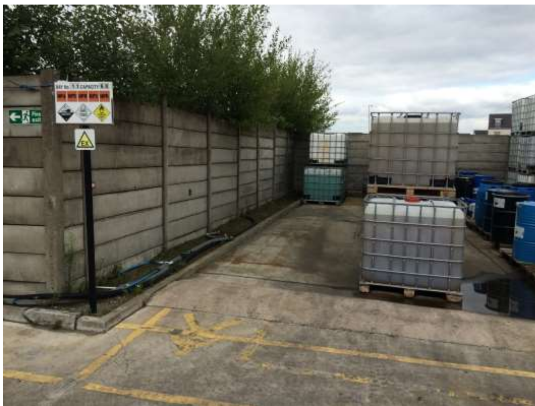
Bay 11 where toxics and oxidisers are stored.
