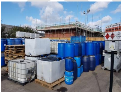
Figure 3 - View from Augean to the block of flats which is still to have a third floor added
