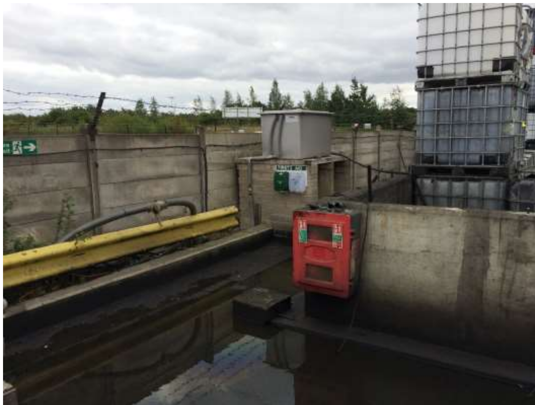
Site eastern boundary
