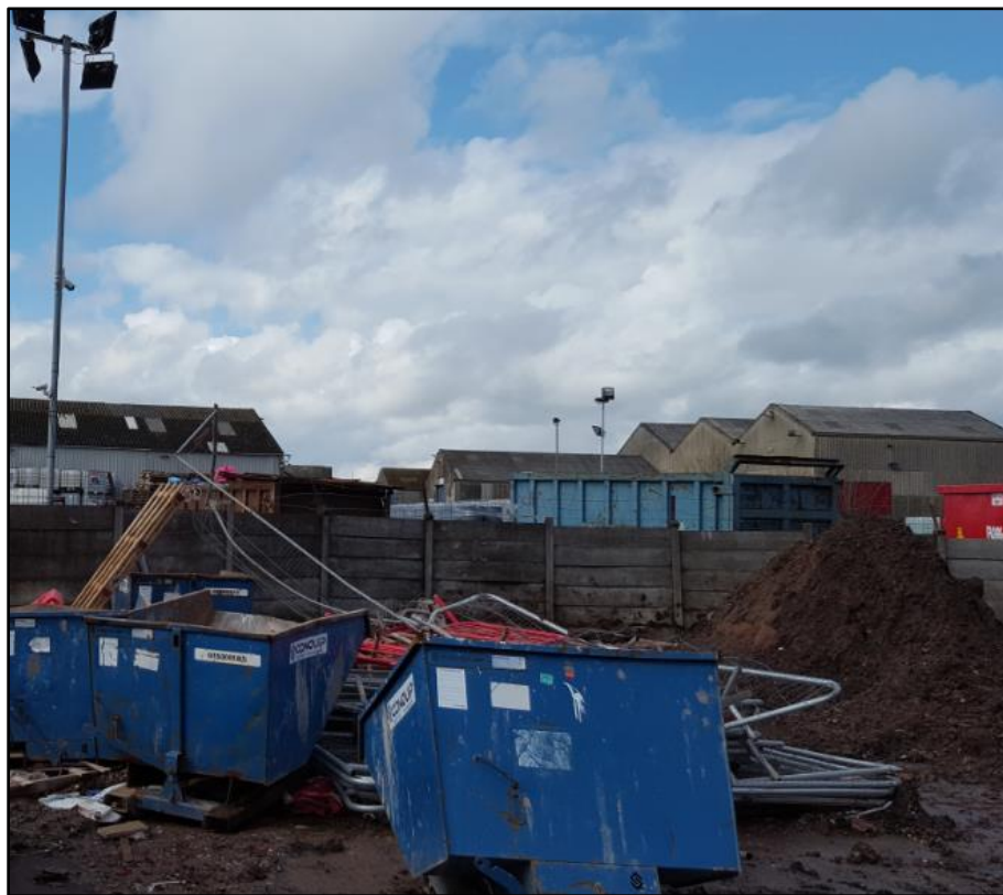
Concrete acoustic fence near vehicle parking spaces
