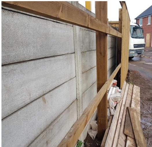
Figure 8 - The gap between the acoustic fence and the concrete barrier
