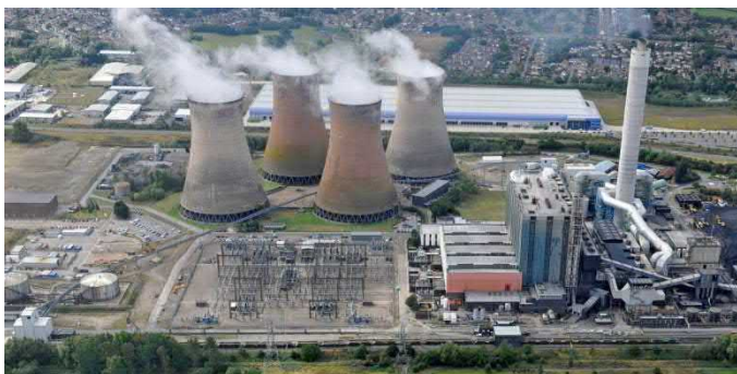
Demolition of Rugeley Power Station began in 2019
