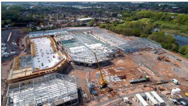
Steelworks for McArthurGlen Designer Outlet nearing completion
