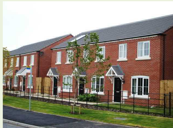
New Houses, Bridgtown
