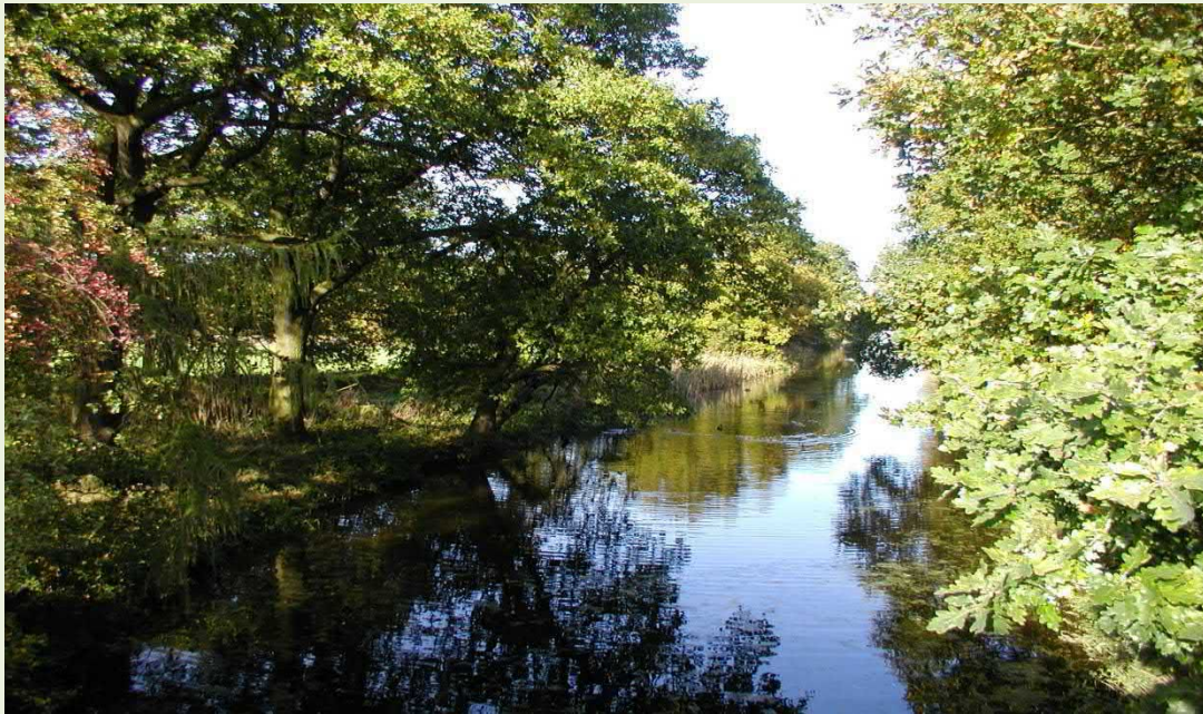
Cannock Extension Canal
