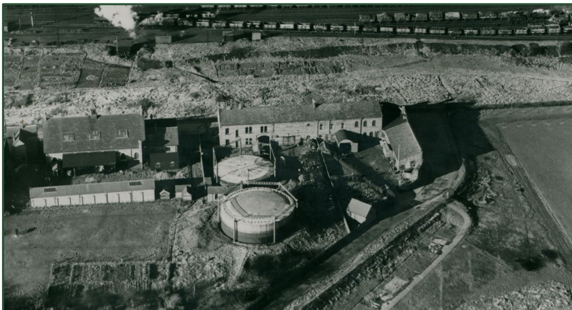
Figure 2: Hednesford Gas Works (courtesy of the Museum of Cannock Chase).
