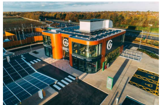
Figure 38: GRIDVOLT charging hub
