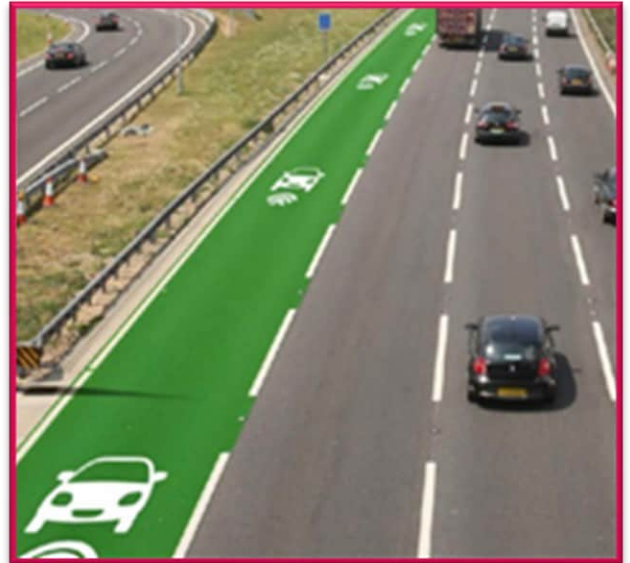
Figure 39: Wireless in road charging
