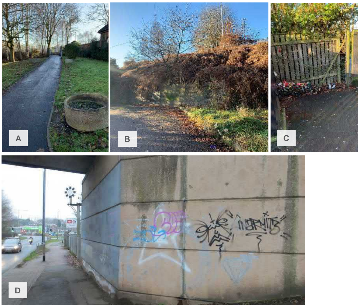
Figure 2-12 - Unattractive Features of the Current Cannock Station.
