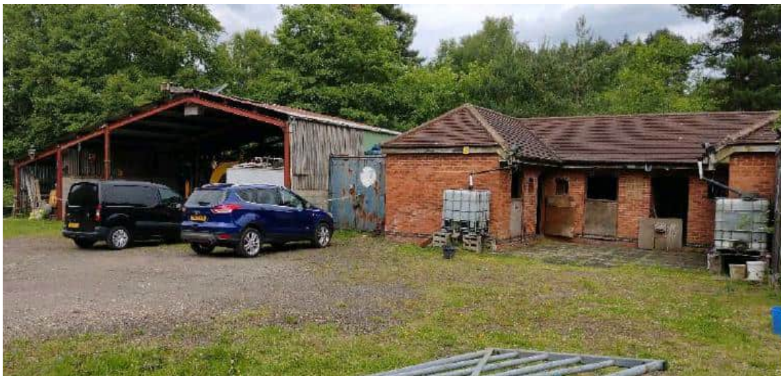
Figure 1: View from the front of the stable building to be demolished (right hand building), left hand building is to be retained
