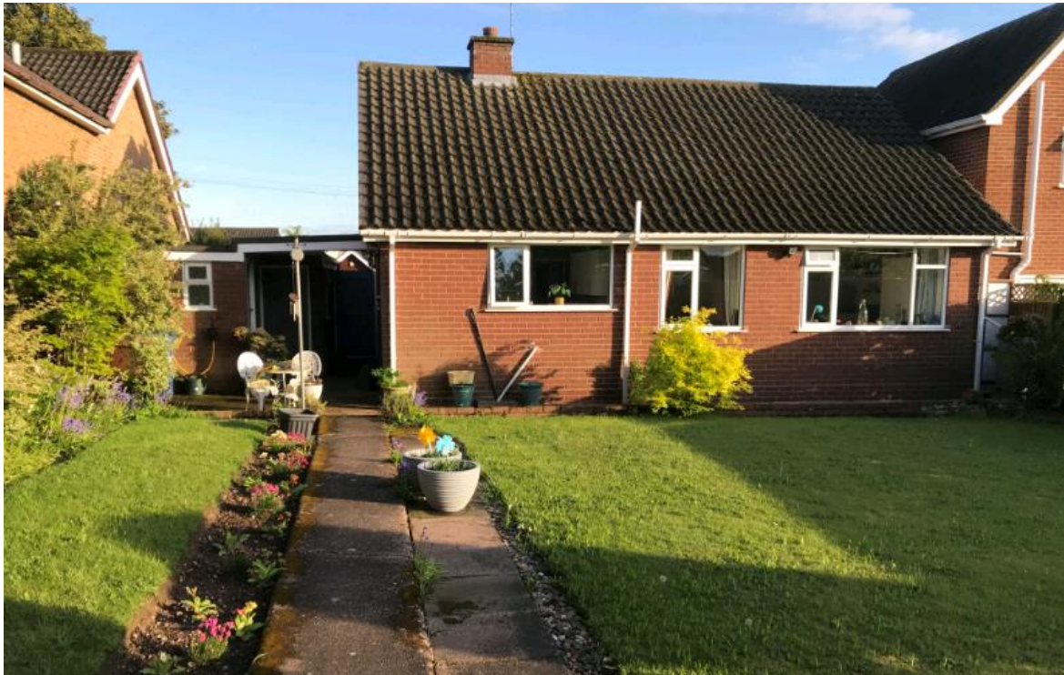
Figure 4: Rear elevation of existing property
