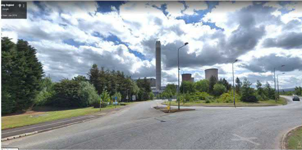
As Existing: Google StreetView along Power Station Road looking East towards the Western Gateway and site entrance
