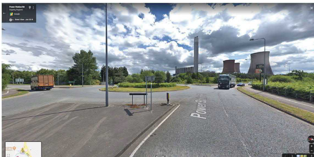
As Existing: Google Street View along Power Station Road looking East towards the Western Gateway and site entrance
