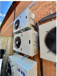
Site photographs of Air conditioning units condensing units and relationship to adjacent building
