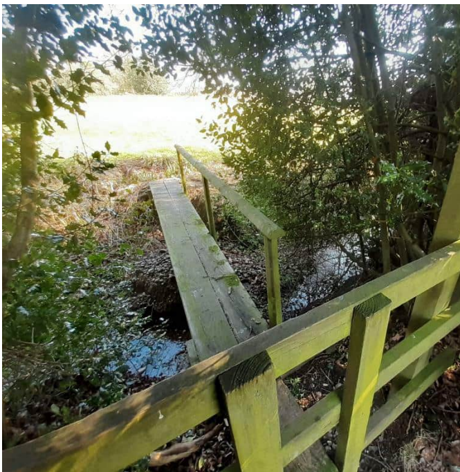
Crossing Shaw Brook on public footpath CW4
