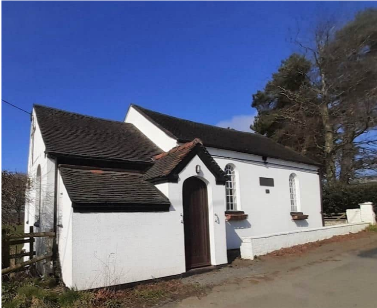
Cannock Wood Methodist Church
