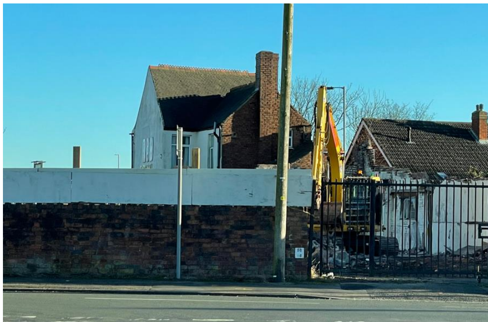
Figure 3: Main view of the site from the rear
