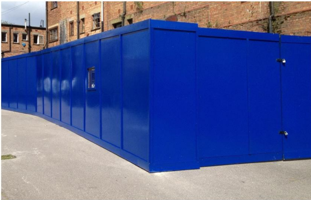
Figure 4: Extract from Demolition Method Statement showing the type of hoardings to be erected around the site
