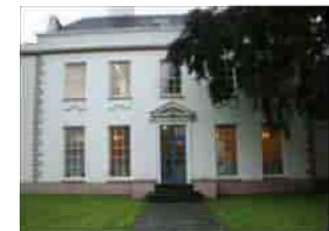
Landmark 4- Listed College Building
