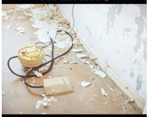
Excessive use of steam strippers can lead to severe damage to plaster wall and ceiling finishes.
