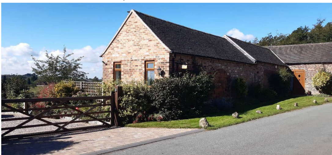
Park Gate Barn
