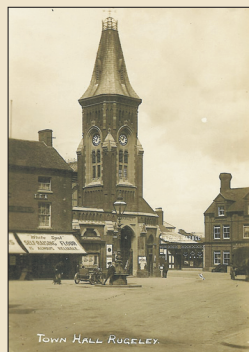
The clock tower is all that is left of the Town Hall of 1878.
