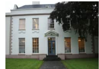
Landmark 4- Listed College Building
