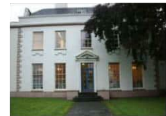
Landmark 4- Listed College Building
