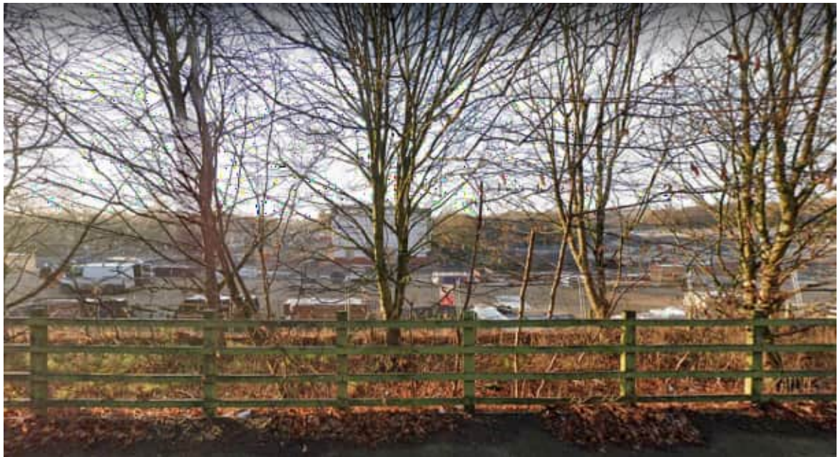
Figure 3.3: View of Crematorium being constructed taken from Cannock Road, November 2020
