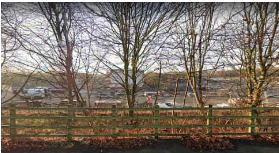
Figure 4.1: View of Crematorium being constructed taken from Cannock Road
